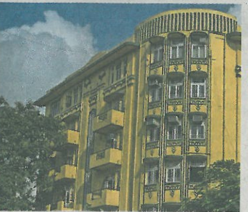
Classic architecture in Mumbai, from top: the Soona Mahal building; the New India Assurance building, which is almost classical in its details; sculptural reliefs that idealize Indian workers on the Assurance building; and Shiv Shanti Bhuvan at Oval Maidan.
